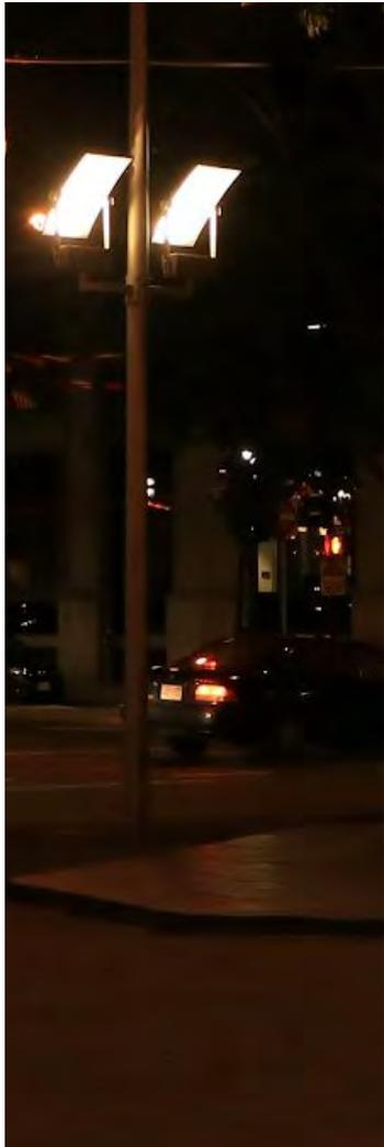
Currently, the only permanent lighting in the 12,000 sq. ft. central plaza is around its perimeter, where 8 poles are mounted with 2 lights each. The lights are directed UP onto diffusers that are supposed to reflect the light onto the area below. In actuality, this system fails to provide ample illumination.
